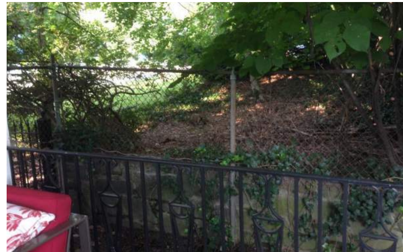
Fig. 4.1.7 - Existing perimeter fence
