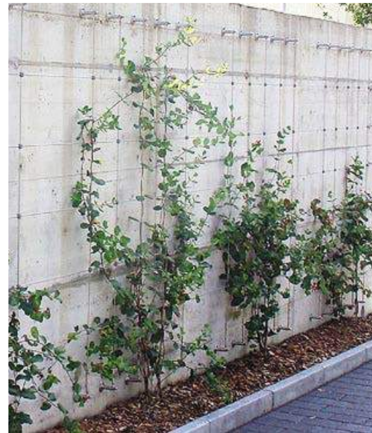
Fig. 2.1.5 - Precedent Image - cable green facade system
