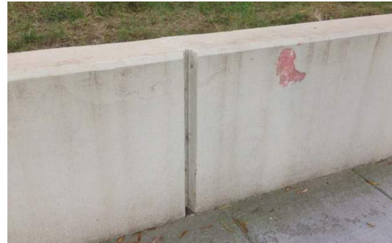
Fig. 4.1.3 - Retaining walls along 34th Street.
