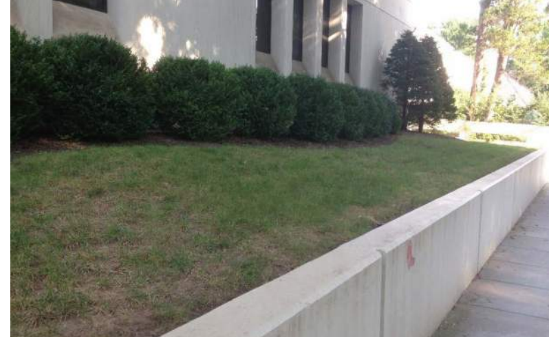
Fig 4.1.2 - Retaining walls along 34th Street.
