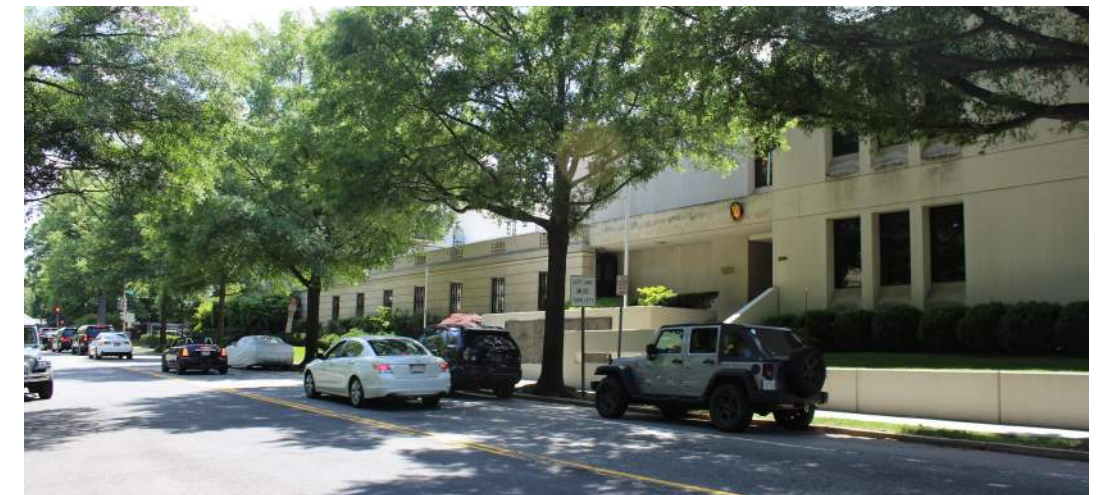
Fig. 4.4 - Chancery facade along 34th Street
