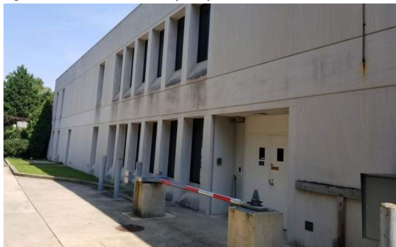
Fig. 4.1.8 - Existing public alley facade
