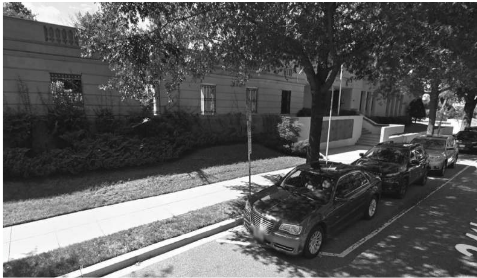
Photo of Existing
