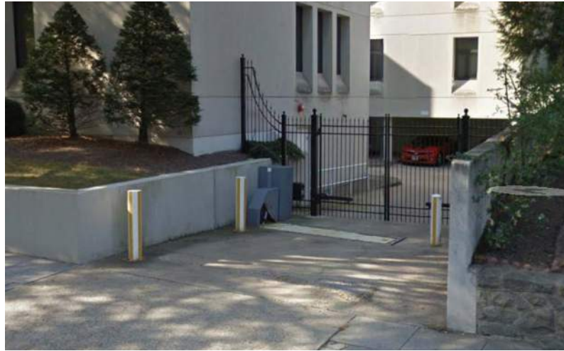
Fig. 4.1.4 - Existing swing arm gate and garage driveway
